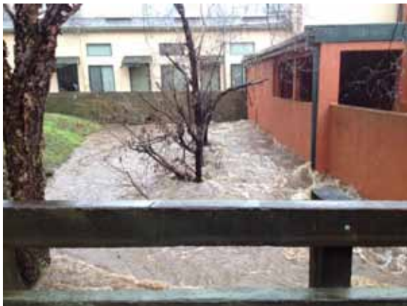
Flooding in Downtown Mill Valley after a rain storm, February 2014
