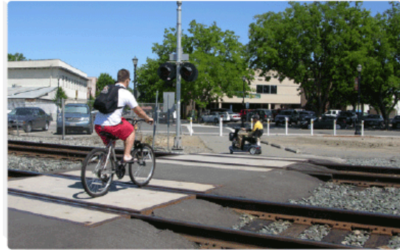
Interim improvements make Dixon crossings safer.
