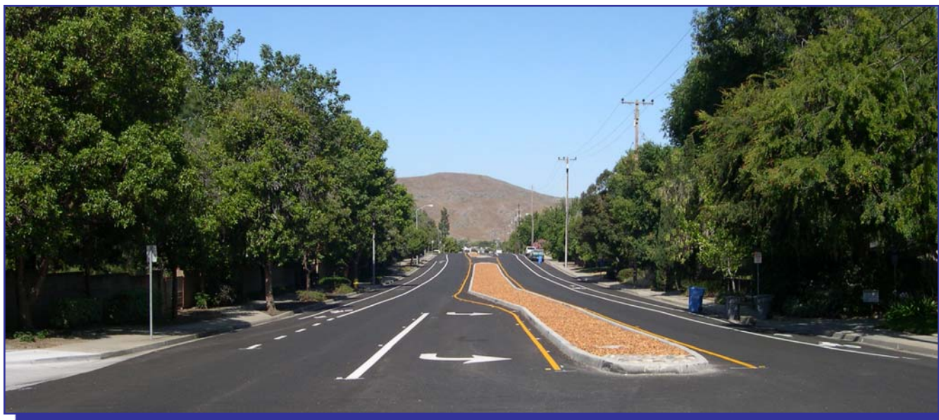
South Street, San Luis Obispo (State Route 227) Recent streetscape and road diet from four lanes to two lanes includes bike lanes, median, and left turn pockets.
