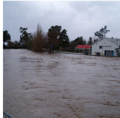
December 2017 high water at top of levee in East Palo Alto.
